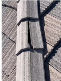
Tile damaged at rear roof hip
