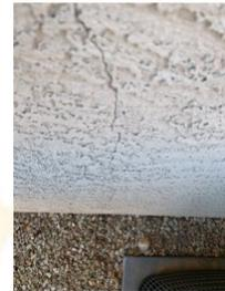
Advise caulking at moderate size stucco crack at Eastside and your AC unit
