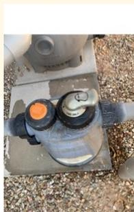
Large leak at top of chlorinstructor at pool equipment
