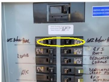
Two upper 20 amp circuit breakers were tripped. Reset OK. For outlets below panel.
