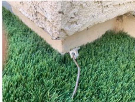
Bond wire not connected to base of stucco wall at rear patio
