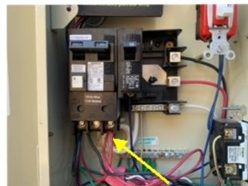
Wiring improperly doubled at pool sub panel
