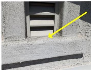
Stucco improperly pitched to pond water at upper gable vent at front roof
