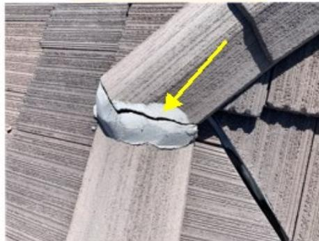
Cracking or separations noted at mortar flashings at rear roof hip
