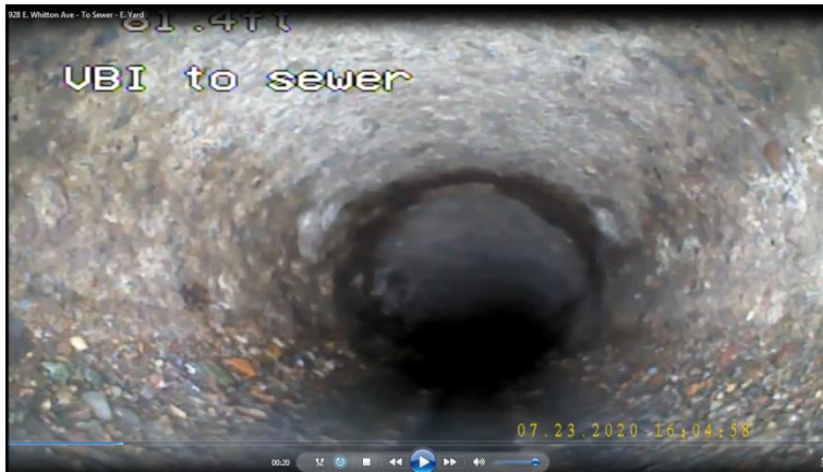
General view of concrete piping
